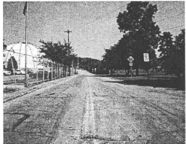
Intersection of Monmouth Avenue and Colerain Avenue, looking east towards Monmouth Overpass (to be improved as part of I-75 Mill Creek Expressway Project).
